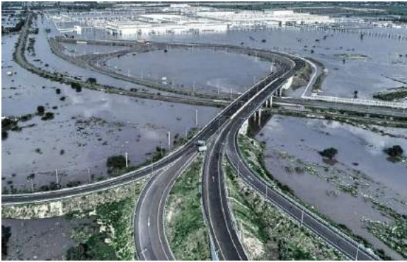
(a) Honda's Celaya Plant after Flood
